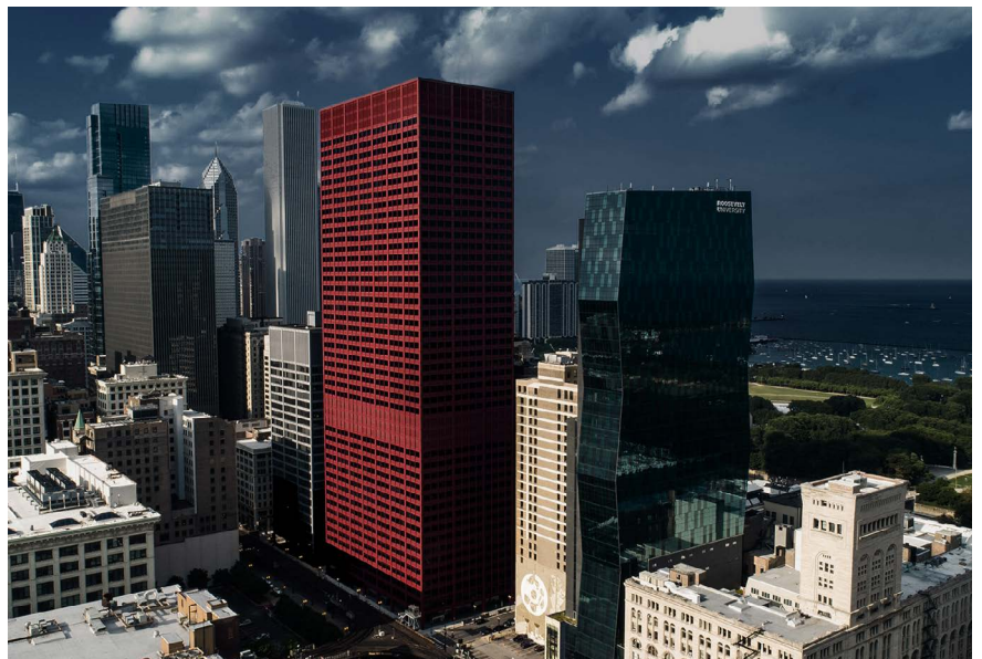
„BIG RED“ PRIME OFFICE TOWER – CHICAGO
